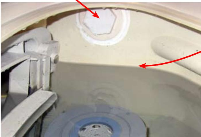
2. Insert Pass-Through Fitting (attached to cell) with wires as illustrated, pull wires into equipment compartment. Tighten Pass-Through Fitting.
